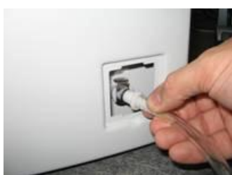
2. Fit hose with barbed fitting to drain
