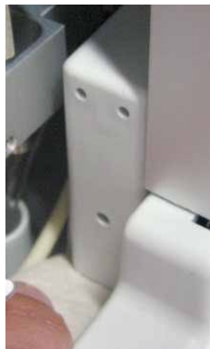
Fig. 37: Drying the leak sensor
